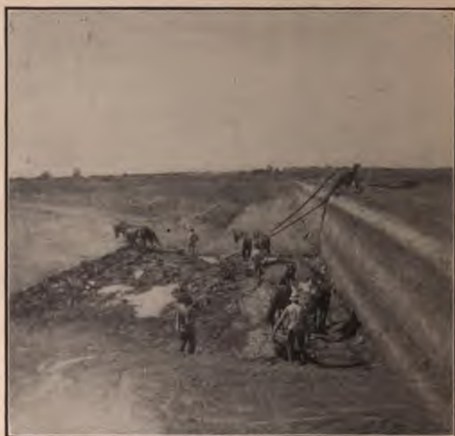
Fig. 56.—Stripping Coal by Scrapers.
